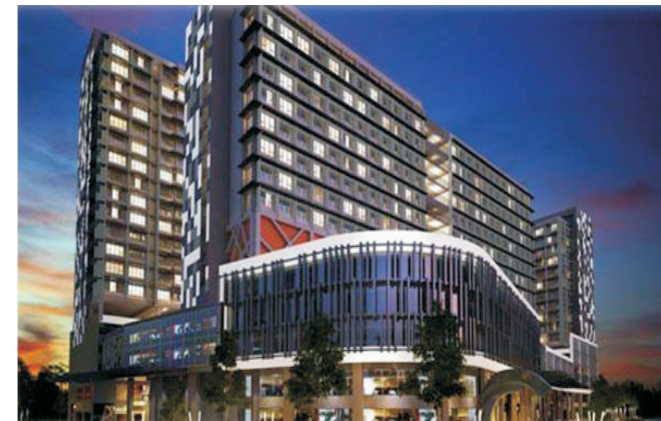
Malaysia Centrestrage Cherish Spring 21st Floor / Station 3.0m/s
