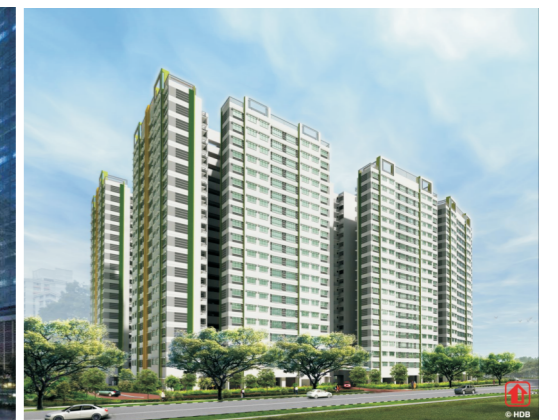
Singapore HDB, Singapore 43 floors / station 4.0m/s
