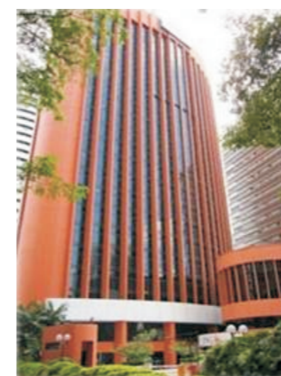
Malaysia Menare ING 22nd Floor / Station 4.0m/s
