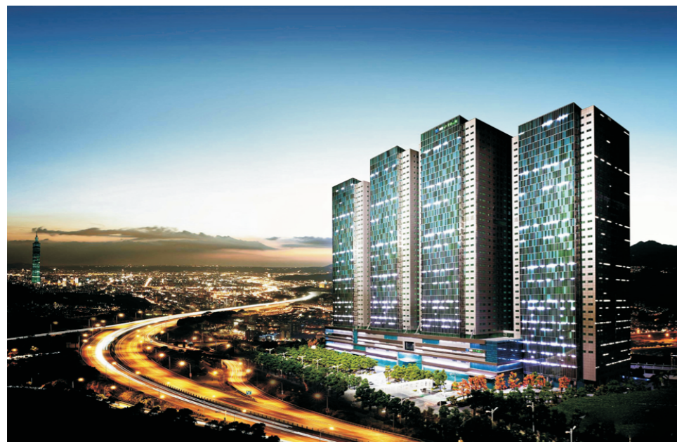
Taiwan's Farglory Cloud U town 42 floor / station 3.5-4.0m/s
