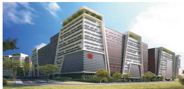
Singapore Industrial Building
